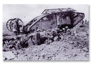
Tanks, like the early British model shown above, enabled armies to travel over uneven ground and barbed wire. Although too slow to be used to full advantage at first, they were devastating against soldiers in trenches.
